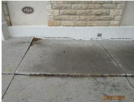
**Downtown Sidewalk.** Staff is contacting potential contractors for repairs to the sidewalk along the south side of Security State Bank. The sidewalk settled several years ago, probably due to poor compaction during the downtown renovation project. Staff would prefer to use a mud-jacking system if financially feasible, to decrease the time of inconvenience in the area.
